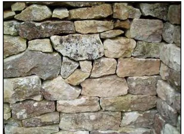
Sometimes the shape of the stones makes this difficult - like a giant jigsaw puzzle. But we try to make all the stones fit tightly together.
