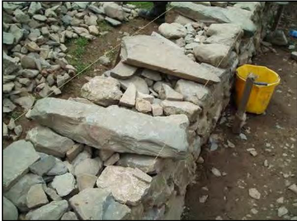
string to make sure the walls are straight and sloping in properly all the way up.
